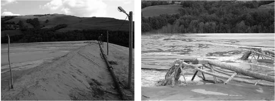
Fig. 1. Decanting pond ‘Valea Salistei’
