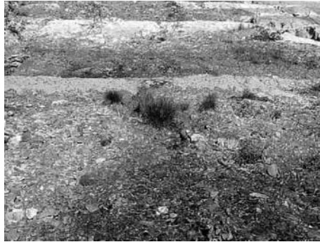
Fig. 3. Water springs on the downstream slope
